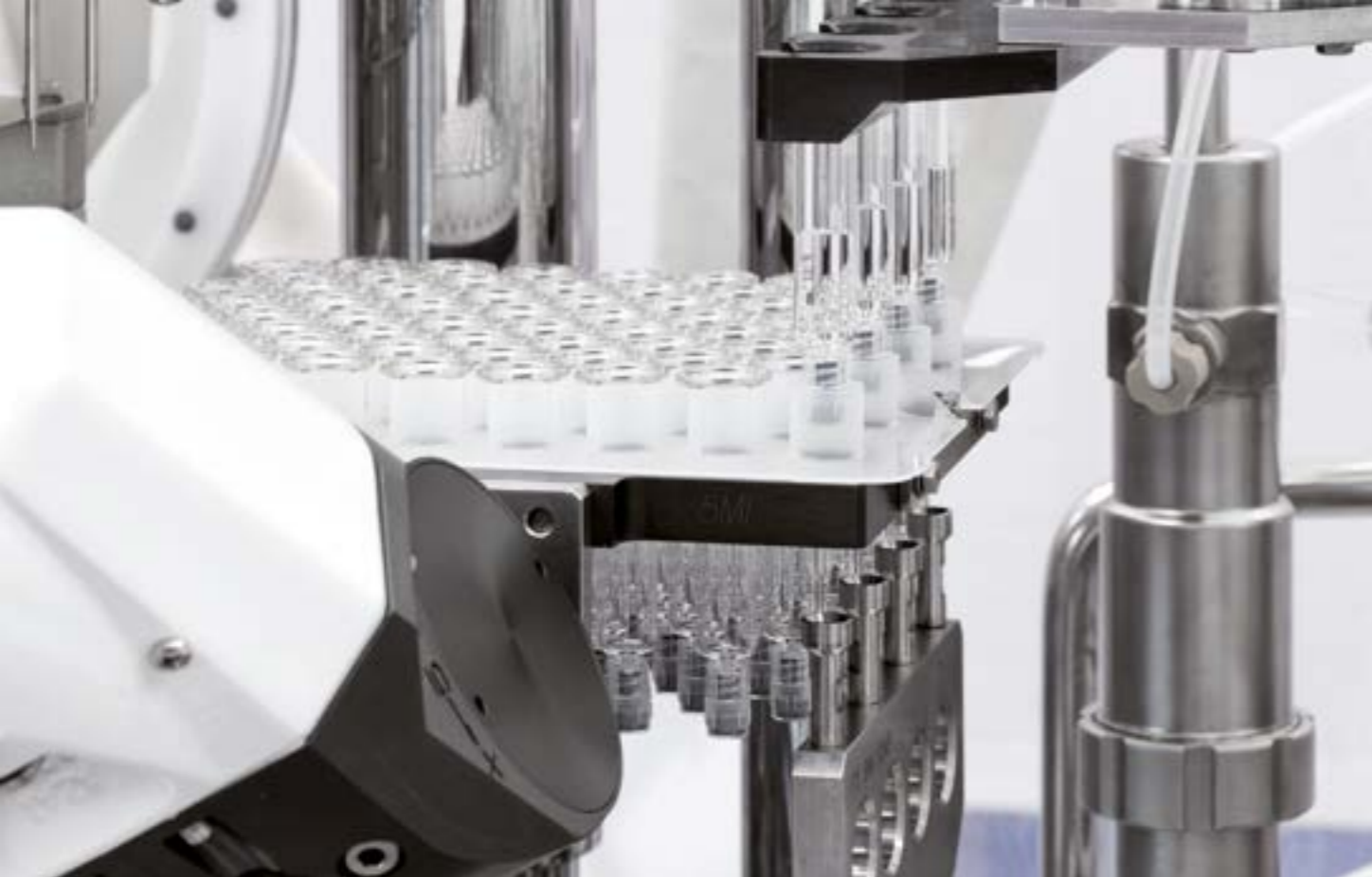
Pre-Filled Syringe robotized filling line and weighing / priming station at CordenPharma Caponago (IT).
